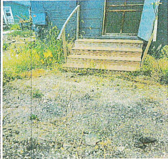
Alley entrance into Werling Building (gravel/dirt)
