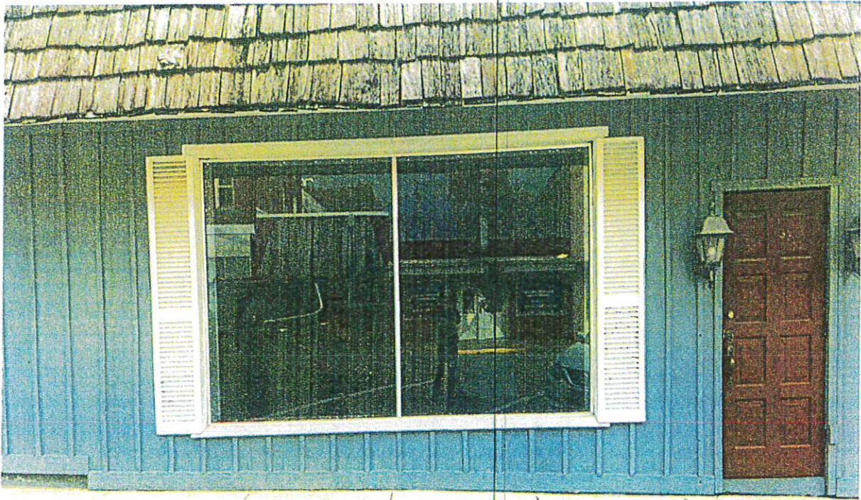
W 5 th Street where glass garage door would be placed
